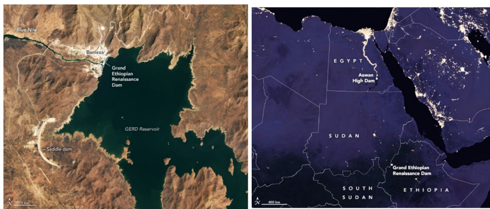
Fig. 3. Construction of the Grand Ethiopian Renaissance Dam (GERD)
